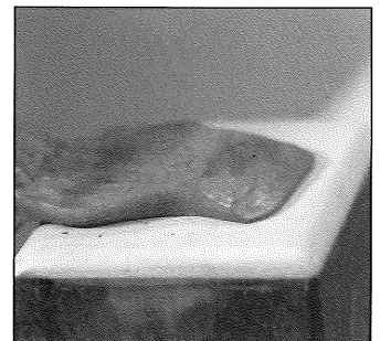
Fig 19. The scarf is tapered and ready for welding
