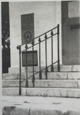
The handrail is at the entrance to the Vereinskirche in Fredericksburg at the center of Market Square. There are six tenoned connections holding this short rail together.
