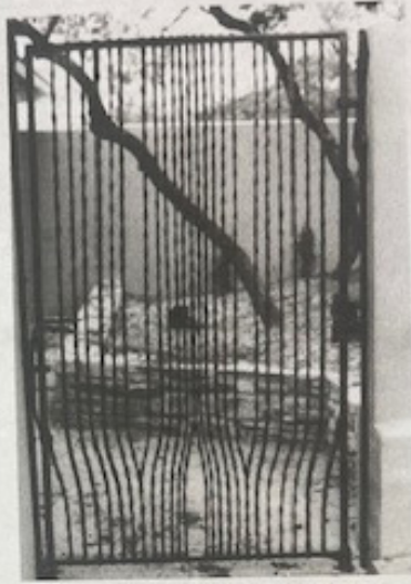
The top rail to a massive garden gate I created 35 years ago. All the vertical stiles are tenoned at the top and bottom.
